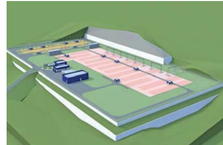
3D representation of the new 400/110/35 kV substation in Lastava.
